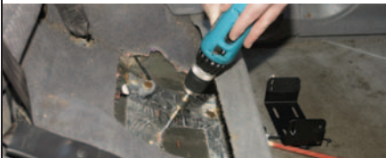
We decided to mount the IC-208H head unit under the rear seat of our '97 Jeep Cherokee, where the factory CD changer would be installed. The carpet already had a cutout, making it easy to remove, and there was a factory heat shield in place to lessen heat transfer from the floorpan.
