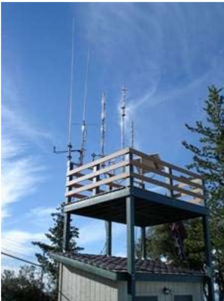
As for the repeater, the stationmaster antenna is in place but not yet connected. It has to be checked out for SWR at the operating frequency and brackets fabricated to accept the transmit and control antennas. The controller is installed and needs some additional tweaking for a better output signal.
